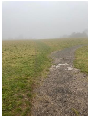
Image shows transition of path from compacted gravel to mowed grass with wheeling's.
